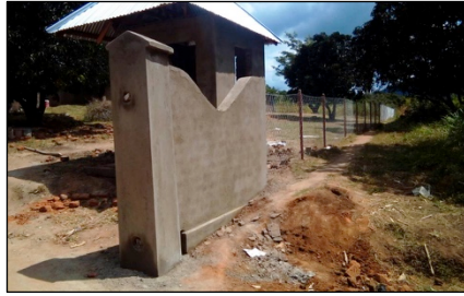
New gatehouse and security fence
