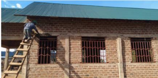
Window grills installed
